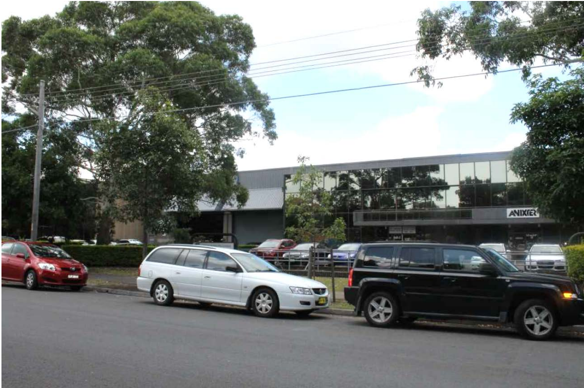
Figure 11: Light industrial buildings at 5-13 Rosebery Avenue
