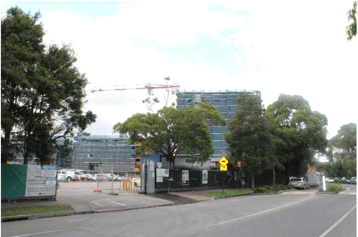
Figure 8: Residential development under construction at 67-97 Dalmeny Avenue viewed from Dalmeny Avenue
