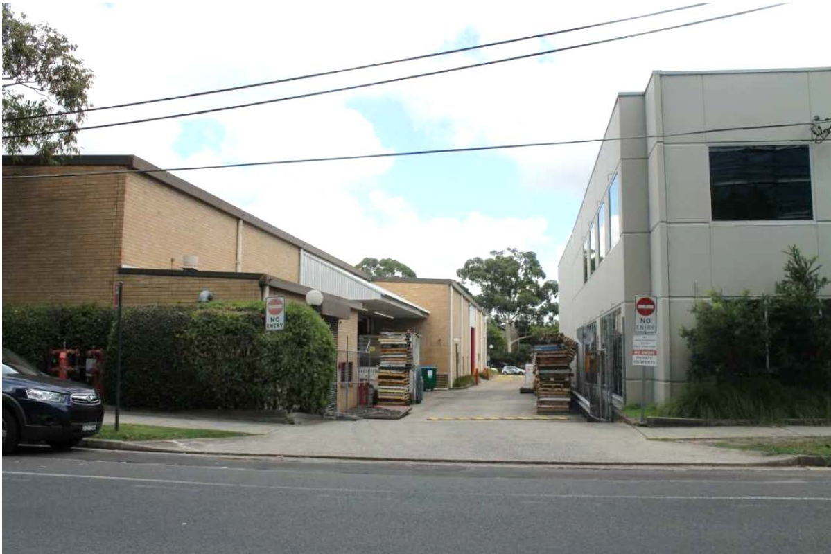
Figure 5: Southern part of the site as viewed from Dalmeny Avenue
