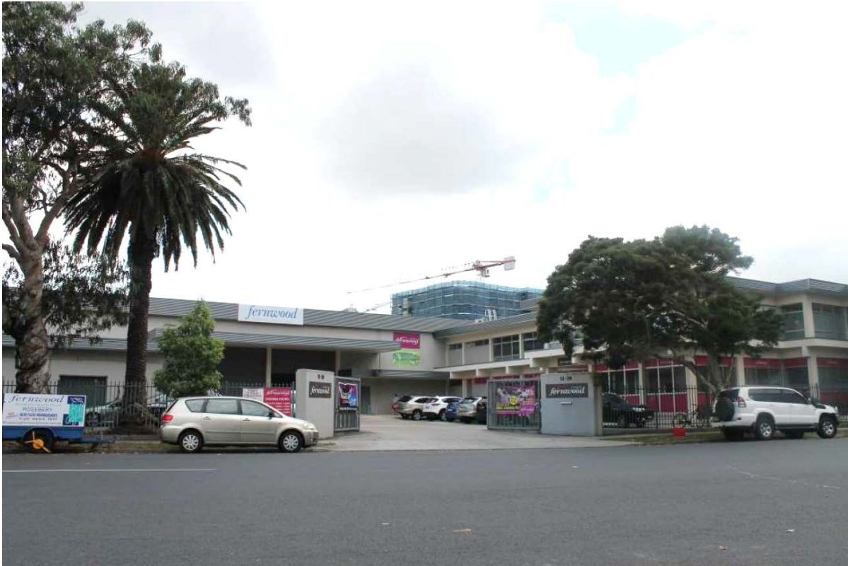
Figure 3: Northern part of the site as viewed from Rosebery Avenue
