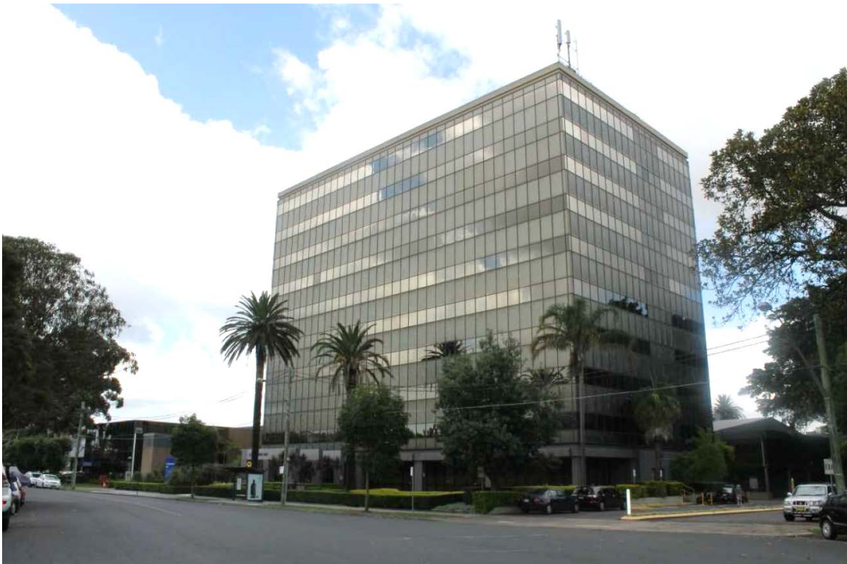
Figure 12: Office building at 5-13 Rosebery Avenue
