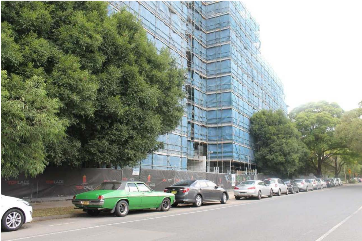
Figure 9: Residential development under construction at 67-97 Dalmeny Avenue viewed from Dalmeny Avenue
