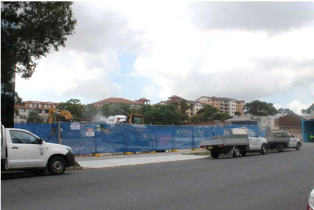
Figure 10: Residential development under construction at 42-60 Rosebery Avenue and 94-102 Dalmeny Avenue
